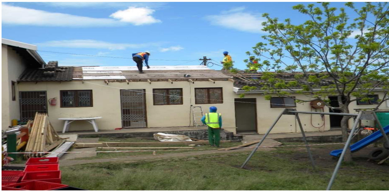
The Building work being carried out at Gozololo
